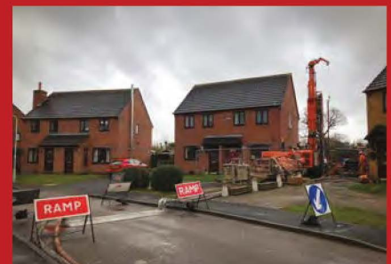
Retrofitting ground source heating as part of a domestic housing installation
